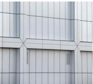
The cladding of the projections attributing the facade its characteristic structure required special customised production. Hence, AGROB BUCHTAL not only designed special panels and cross-sections: assembly was also based on an individual and detailed solution featuring a combination of K20 clamps and K20 system profiles. Based on detailed drawings, the arrow-shaped panels for the intersections were cut precisely in the factory in various sizes.
